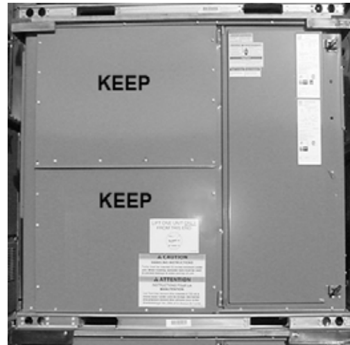
Figure 20: Save Side Panels For Economizer Hood Tops
