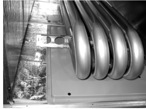
Figure 19: Discharge Panel In Place
